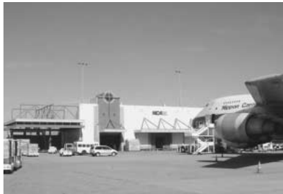
The San Francisco Branch warehouse
